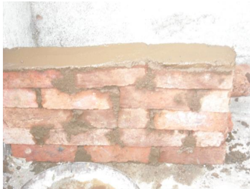
Fig 2. Side view of a section of cavity wall constructed
