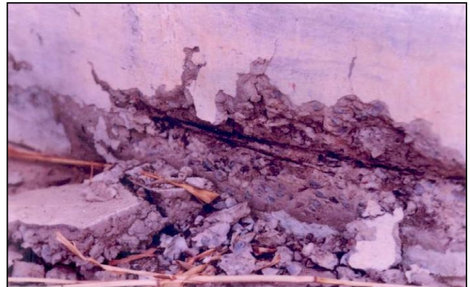
Fig. 13. Shaft at ground level
